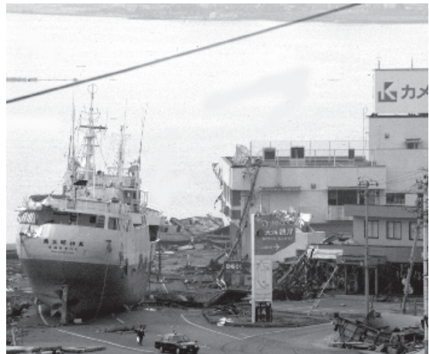
Myojin-Maru stranded ashore by tsunami (Photo by Taikai Kumagai)
